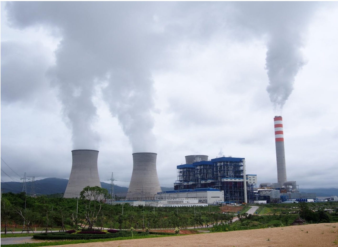
Photo 3: Hongsong coal mining and power plant in Xayaburi province, Lao PDR.
